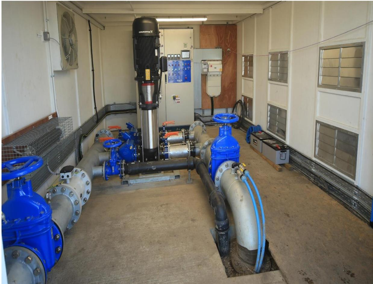
This valuable water resource that is captured, is then returned back in land, via a pipework network to a combination of existing and new winter storage reservoirs. The pipeline consists of two 200mm PVC pipes laid next to each other in a common trench. Release of water to reservoirs is controlled through a series of stations that have remote control valves and flow recording, connected to a portal that allows access to all farmers.
