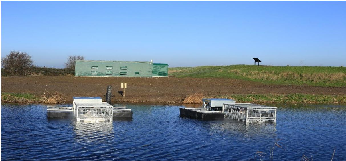
Quality of water coming into the system is monitored by a 7-way sonde that allows a range of water quality parameters to be monitored and the pumps to be stopped if thresholds are reached. Because of the proximity to the sea the biggest concern is saltwater ingress. However, the only concerns to date, have come from elevated conductivity levels related to salt that is spread on the roads during icy conditions, making its way into the drainage water.
